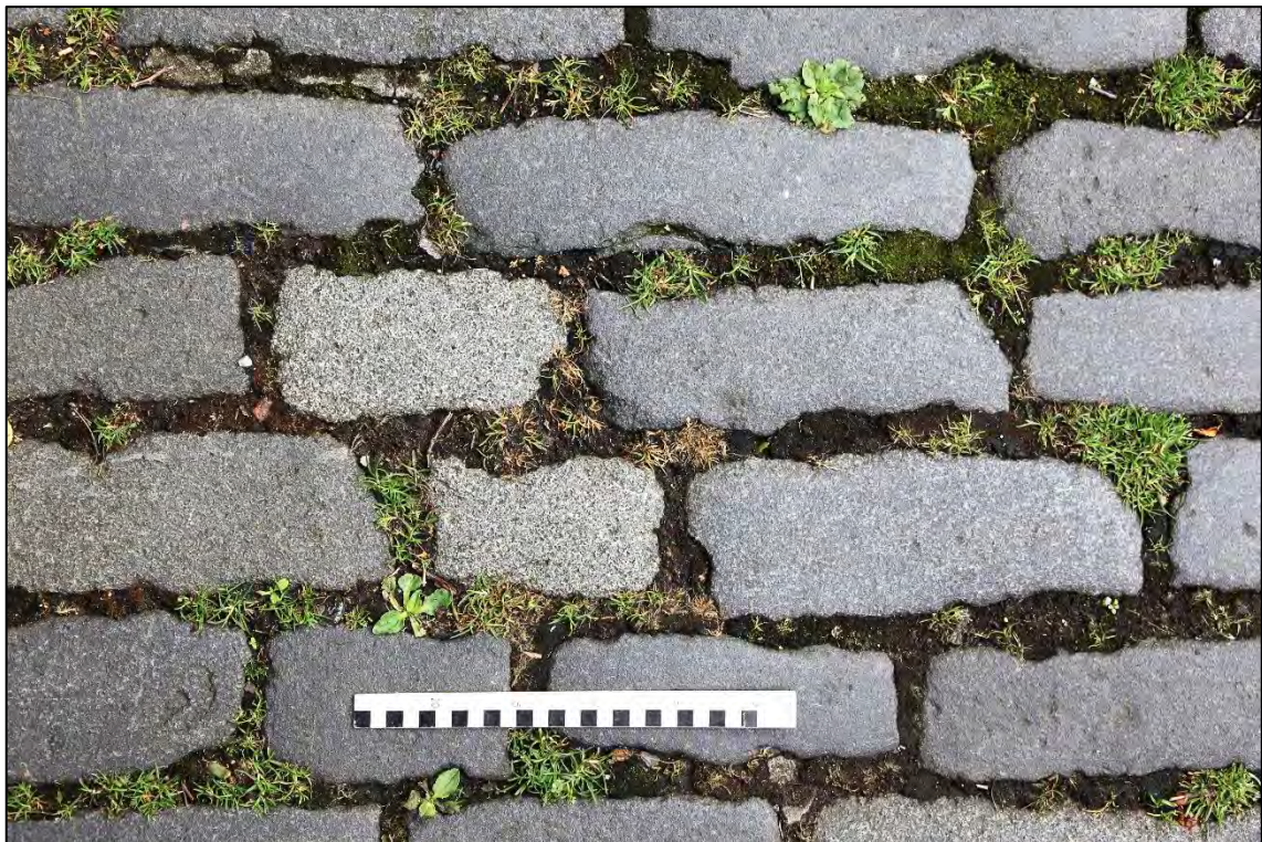
Figure 1 Typical character of a traditional setted street in Edinburgh
